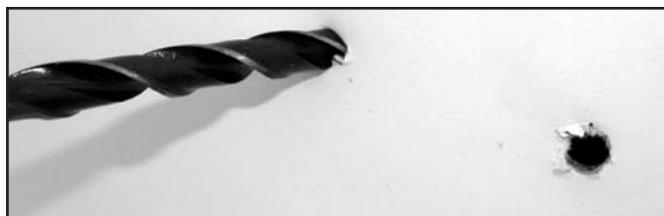
**8. Now (heart pounding) drill the holes. We suggest not center punching, but, instead, starting with a small (1/8" or so) super-sharp bit. Once the holes have been drilled, it's a good idea to brush-apply a little primer to the exposed bare metal surfaces.**
